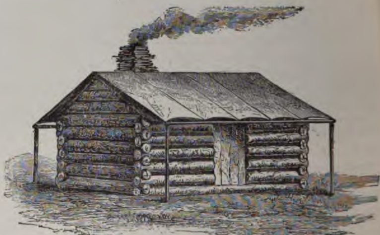
FIG. 196.—Log hut with canvas roof. ( Smart. )
